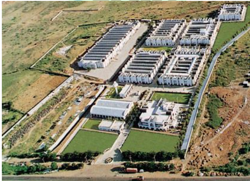
Plastic Park, Jalgaon
