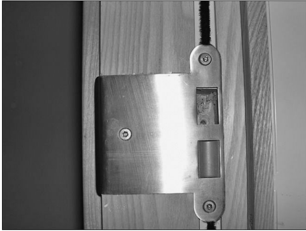
FIGURE 8.2 A strike plate helps prevent the bypassing of locked doors.
