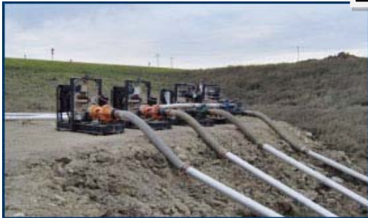
Drain laying for transport of fluids
