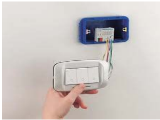
Installation of electronic device
