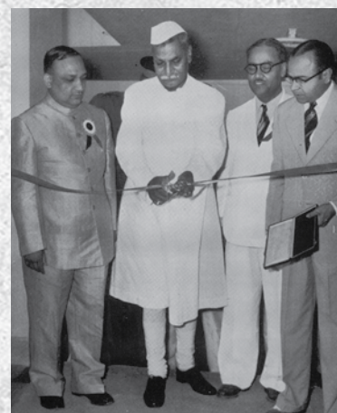
Rashtrapati opening the Building address.
