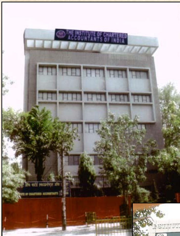
ICAI Building in the year 1999 – At Golden Jubilee
